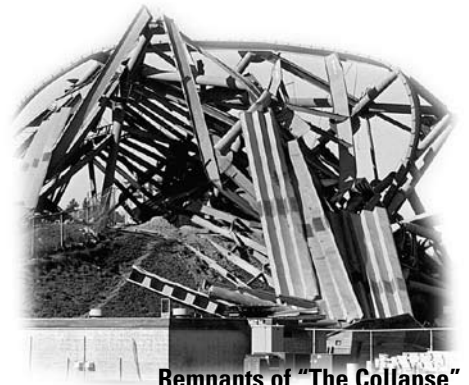
Remnants of "The Collapse"
